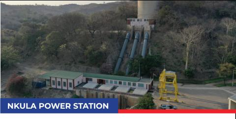
Nkula Power Station is the first major hydro power station in Malawi. It comprises of Nkula A with 3 machines, each rated 11.7MW, and Nkula B with 5 machines, each rated 20MW. The last machine at Nkula A was commissioned in 1966 where as the last machine at Nkula B was commissioned in 1992. The total generation capacity is 135.10MW as detailed below:
